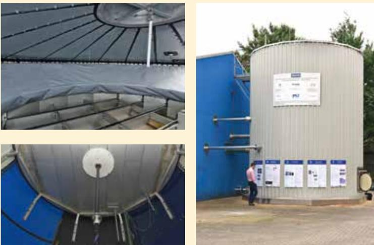
**Fig. 3** Top left: The floating roof in the roof area is flexibly sealed. For insulation the segments are filled with PU bulk. The outer layer form accessible XPS thermal insulation panels. Bottom left: The upper diffuser is integrated in the floating roof. Its form has been specially optimised. Right: The 100 m<sup>2</sup> demonstrator in Nortorf has been extensively tested for more than one year.
