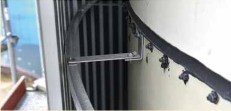
**Fig. 2** Structure of the storage tank wall: The cladding panel is connected to the screwed segments via thermally decoupled stainless steel strips. The spaces in-between are insulated with a polyurethane bulk.
