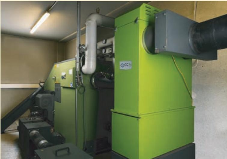
Fig. 3 A 100-kW fine dust filter in the field trial
