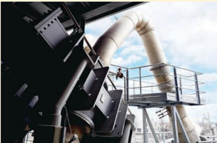
**Fig. 3** Above: The lime moving bed leaves the reactor, the ash and pollutants are then filtered out. Below: Raw gas pipes with safety discs.
