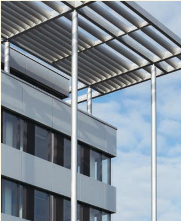
**Fig. 3** Static solar protection on the mathematics building in the south campus of the Karlsruhe Institute of Technology
