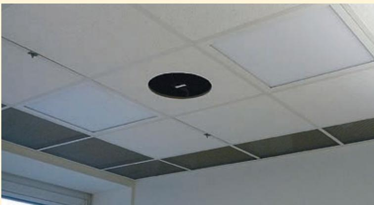
**Fig. 4** Grid ceiling with integrated, workplace-specific fan: As well as the fan, two LED lights are installed. Extended metal mesh panels are installed in the edge area of the ceiling.
