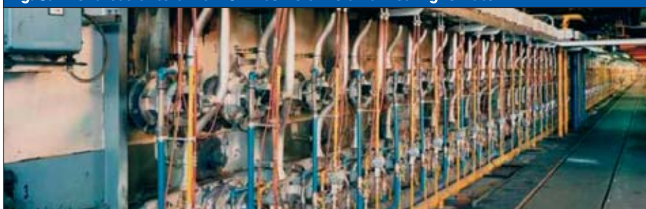
Fig. 5: Hundreds of ceramic FLOX® burners fire an annealing furnace
