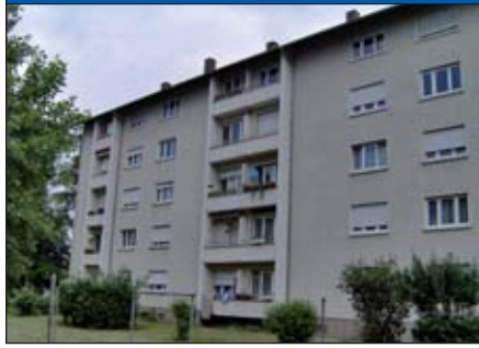
Fig. 4: Typical transom building in original condition
