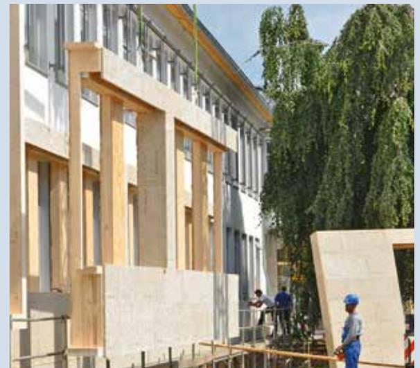
**Fig. 5** Installers fit the prefabricated modules; they are then filled with cellulose.
