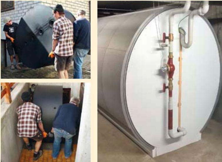
**Fig. 3** Left: Workers carry a storage module through a narrow cellar entrance, Right: UniSto storage tank with thermal insulation made of silver-grey Neopor® shell plates.
