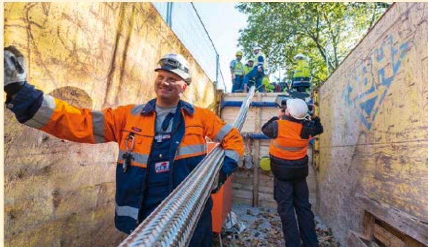
**Fig. 2** Laying the superconducting cable in the inner city of Essen
