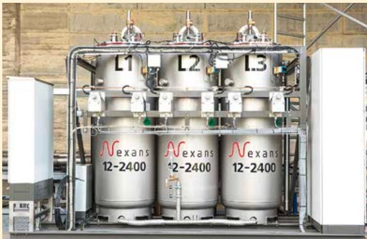
**Fig. 4** The fault current limiters for the three phases are located in separate cryogenic containers.
