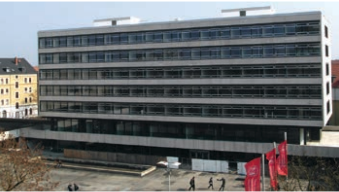
Fig. 1 The „Forum“ building on the central campus: A typical functional building from the era when the universities were established again at the end of the 1960s, which was refurbished in 2014/15
