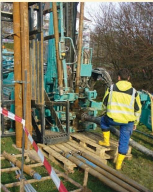
Fig. 5 Installation of borehole heat exchangers beneath an open space in the Sonnenberg-Southwest area.
