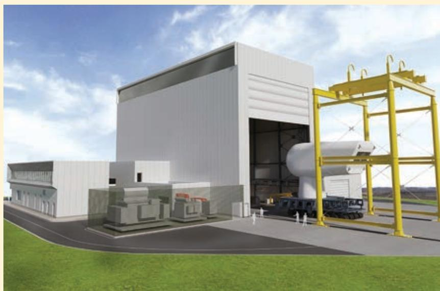
Fig. 2 Simulation: a nacelle is driven on a heavy load transporter into the 30-metre-high testing hall. The yellow gantry crane can raise loads of up to 420 tonnes.
