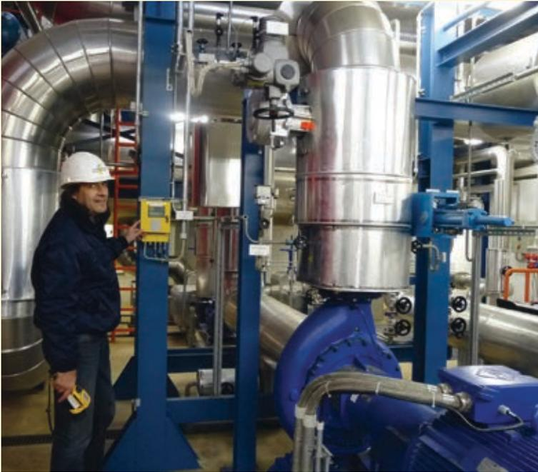
**Fig. 3** Inside the municipal utility company's heat transfer station in Jena: The plant transfers the heat from steam to hot water.
