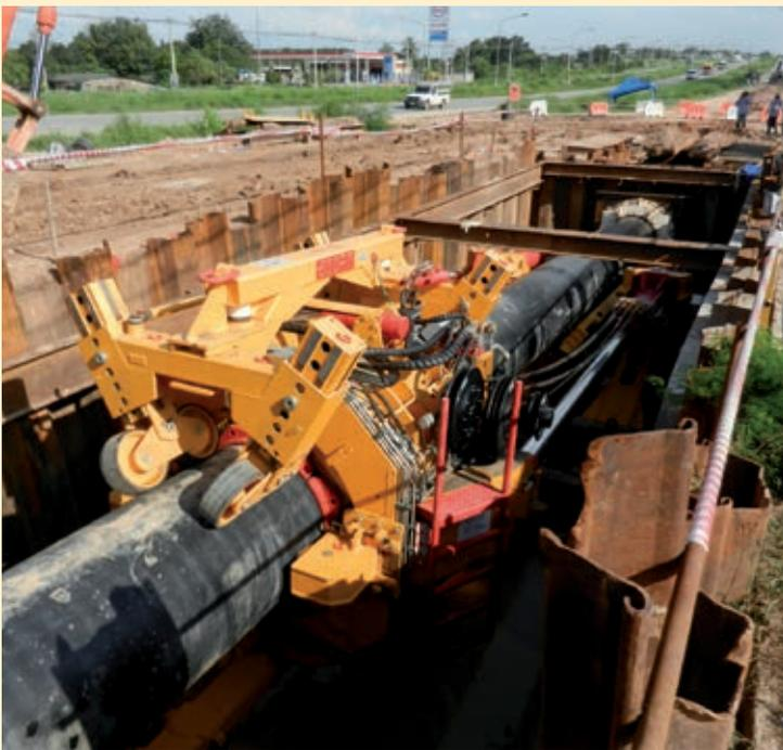
Fig. 4 With up to 750 tonnes of thrust, the so-called pipe thruster lays the pipelines into the horizontally drilled borehole at five-metre increments.
