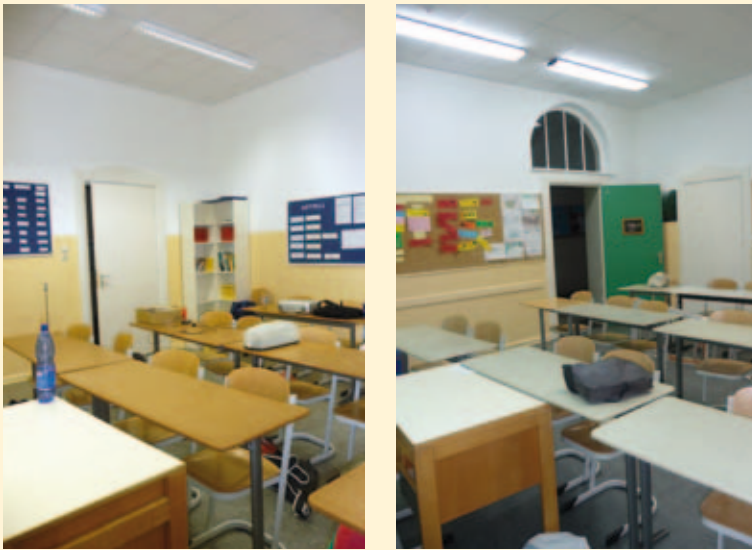
Fig. 2 Lighting situation in the classrooms after installing the optimised lighting and ballast technology: Left the energy efficient and warm white (4,000 K) lighting, right the learn-promoting bluish lighting (6,500 K). Source: TU Berlin
