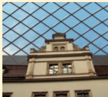
Fig. 6 Residential Palace, Dresden, membrane roof. Architect: P. Kulka, P. Stamborski. Source: Jochen Manara
