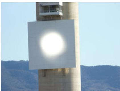
In solar thermal power plants, the solar radiation is focussed on a point (the receiver).
