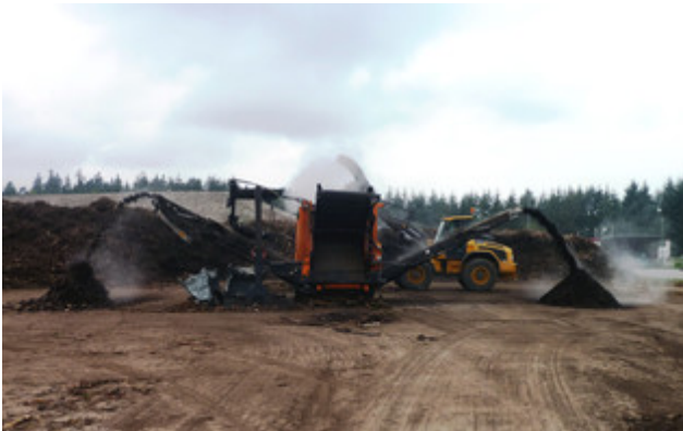
The researchers are investigating how the proportion of fuel and compost fractions as well as the fuel quality of collected green waste varies over the course of the year, depending on different treatment lines and input material.
