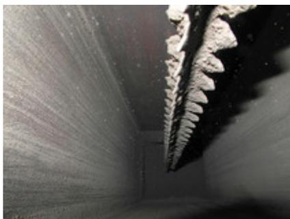
Interior view of the precipitator box: The deposited particulate matter can be seen at the electrodes.
