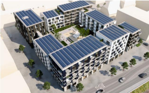
Bèla is the first of six residential/commercial blocks in the Neue Weststadt urban district in Esslingen. The three buildings have 132 residential units. The roof's coverage with a roughly 250-kWp photovoltaic system enables the utilisation of renewable energy that is marketed using a tenant electricity model.
