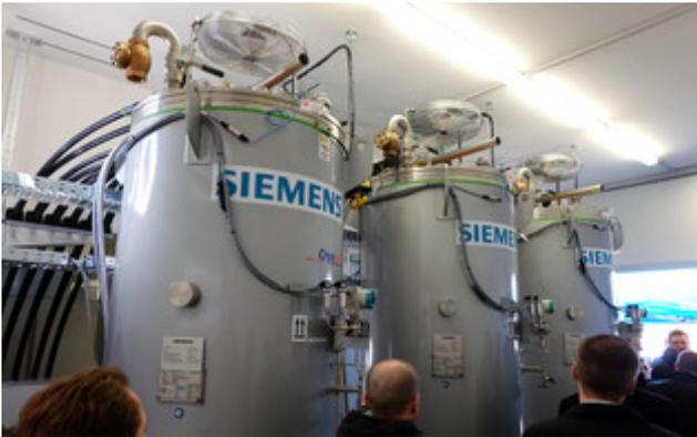
The fault current limiters for the three phases of the electricity grid are housed separately in cryogenic containers. Closed cooling systems ensure the low temperatures. The whole system is so compact that it can be housed in a prefabricated container.
