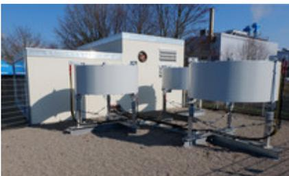
An inductor is connected parallel to the fault current limiter for every phase.
