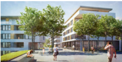
170 new climate-neutral homes are set to be built on the outskirts of Überlingen.
