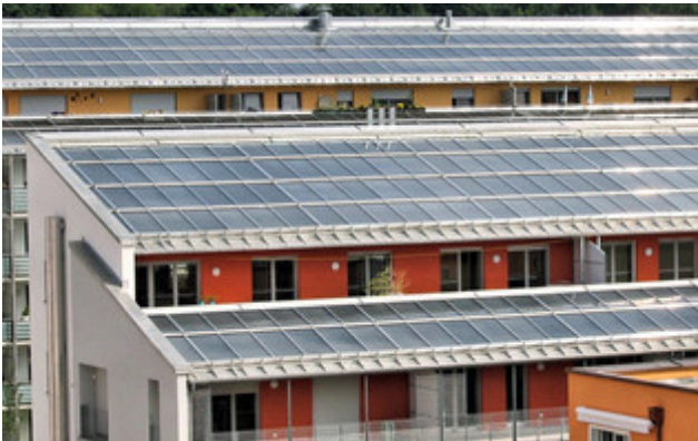
Number of large-scale solar thermal systems in heating networks rising. Photo shows the “Solar local heating district”, the third of four construction phases of the “Ackermannbogen” redevelopment area in Munich.
