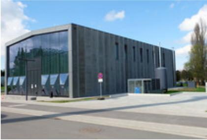
View of the south side of the building: The large window area of the ETA Factory equipped with light control elements allows for the optimal use of daylight in the hall. The external high-temperature vacuum storage unit is to the right of the building.
