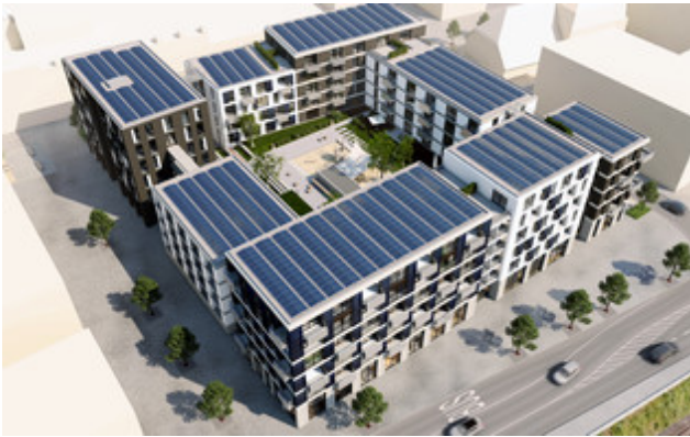
Bèla is the first of six residential/commercial blocks in the Neue Weststadt urban district in Esslingen. The three buildings have 132 residential units. The roof's coverage with a roughly 250-kWp photovoltaic system enables the utilisation of renewable energy that is marketed using a tenant electricity model. © Graf und Graf Architekten
