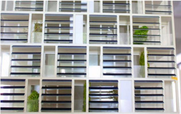
The Smart Green Tower will have a building envelope made of glass/glass photovoltaic modules with Perc cells.
