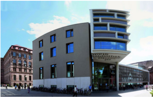
Up to a fifth of the energy costs of municipal real estate can be saved by means of communal energy management. Photo shows the central library in Nuremberg, Germany, consisting of the renovated existing building and a newly constructed elongated block. © Hochbauamt Stadt Nürnberg
