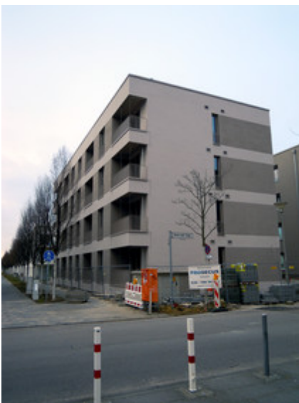
House 3 with the PV system on the roof shortly before completion
