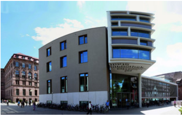
Up to a fifth of the energy costs of municipal real estate can be saved by means of communal energy management. Photo shows the central library in Nuremberg, Germany, consisting of the renovated existing building and a newly constructed elongated block. © Hochbauamt Stadt Nürnberg
